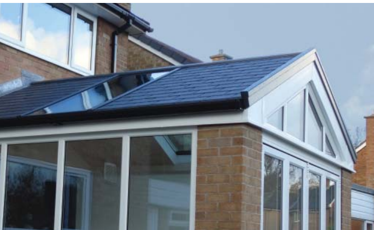
UltraRoof380 allows the installation of full height rectangular glass panels
