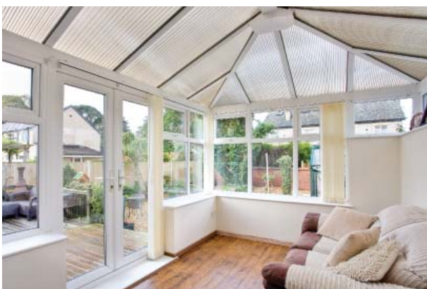
BEFORE the transformation with a tired polycarbonate roof.
